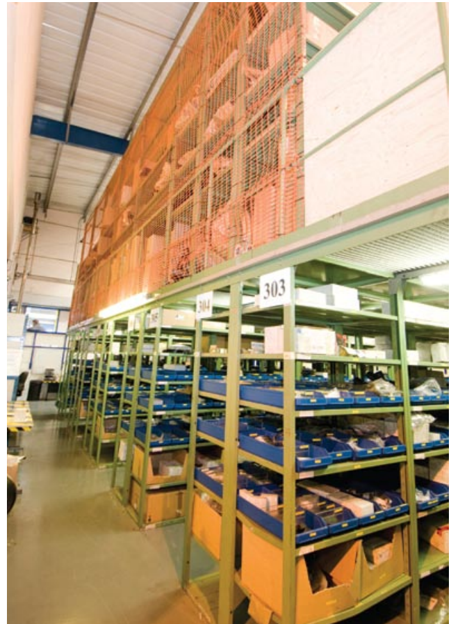
Figure 87 Stable racking with protection against falling objects
