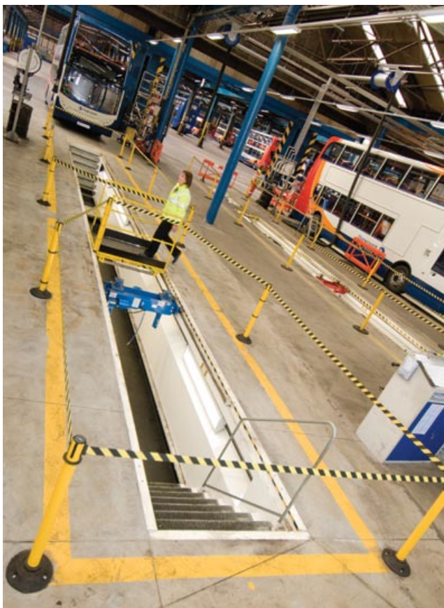
Figure 63 Moveable bridge allowing access across middle of pit
