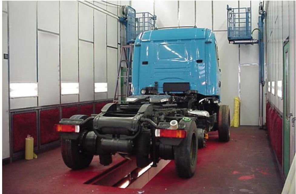
Figure 17 A spray booth for commercial vehicles with moveable gantries provides safe access for spraying at height
