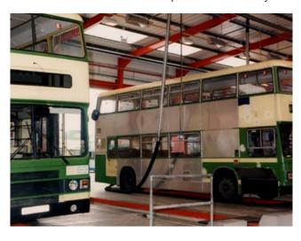
Figure 3 Bus using a tailpipe exhaust extraction system to control emissions
